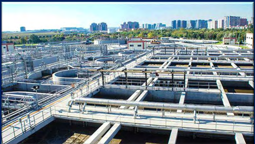
Atakoy Wastewater reuse Plant - Aeration Tanks II Stage
