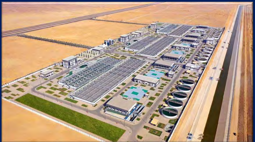
Bahr Al-Baqar Wastewater Reuse Plant-Egypt.
