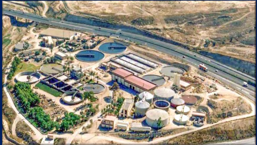
Rincón de León Wastewater Reuse Plant. Alicante, Spain.
