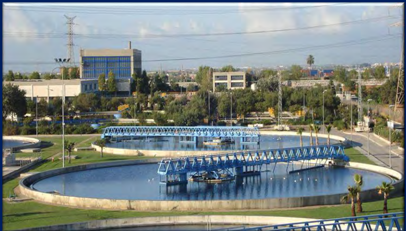
Pinedo Wastewater Reuse Plant – Valencia, Spain.
