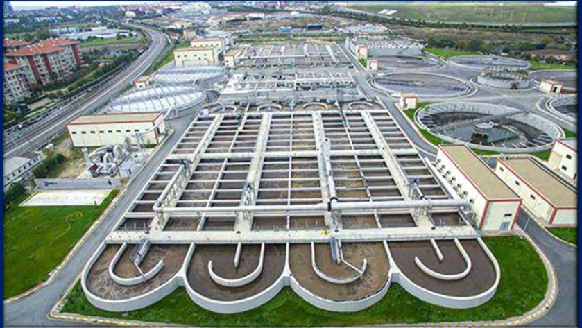
Atakoy Wastewater Reuse Plant – Istanbul, Türkiye.
