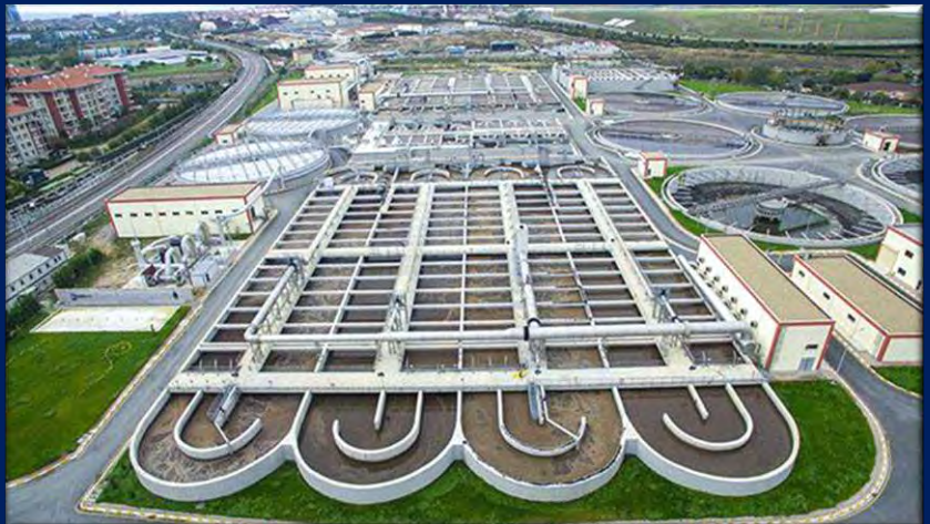
Atakoy Wastewater Reuse Plant – Istanbul, Türkiye.
