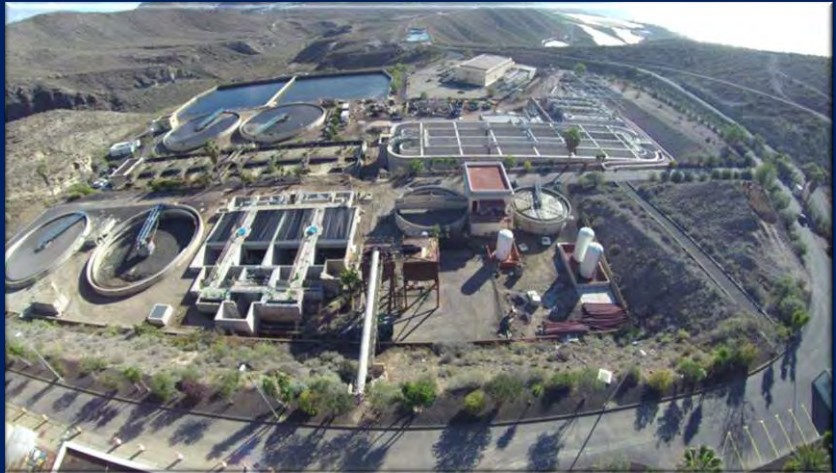
Adeje-Arona Wastewater Reuse Plant. Tenerife, Spain.
