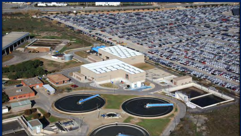
Tarragona Wastewater Reuse Plant. Tarragona, Spain.
