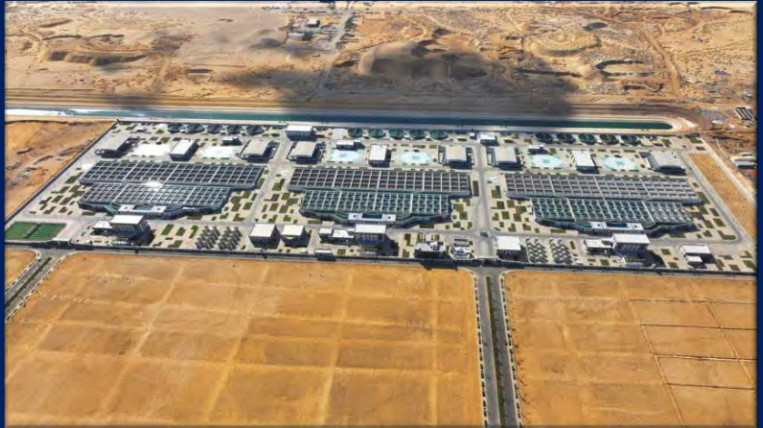
El Hamam Wastewater Reuse Plant–Egypt.
