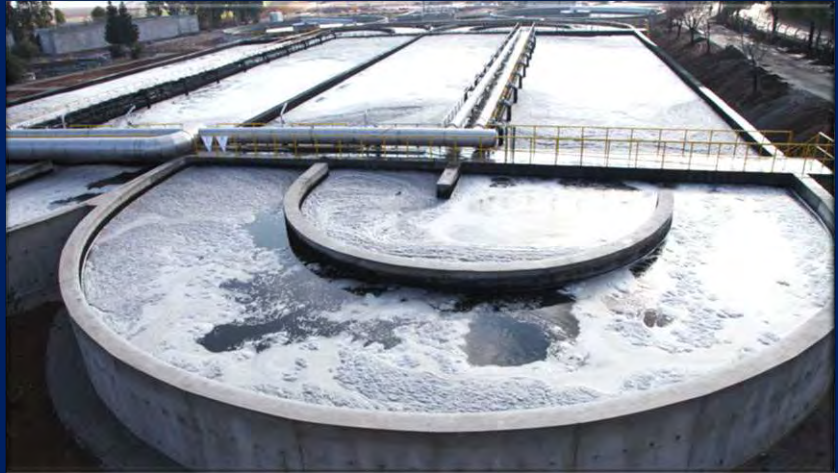
Akhisar Wastewater Reuse Plant – Türkiye.
