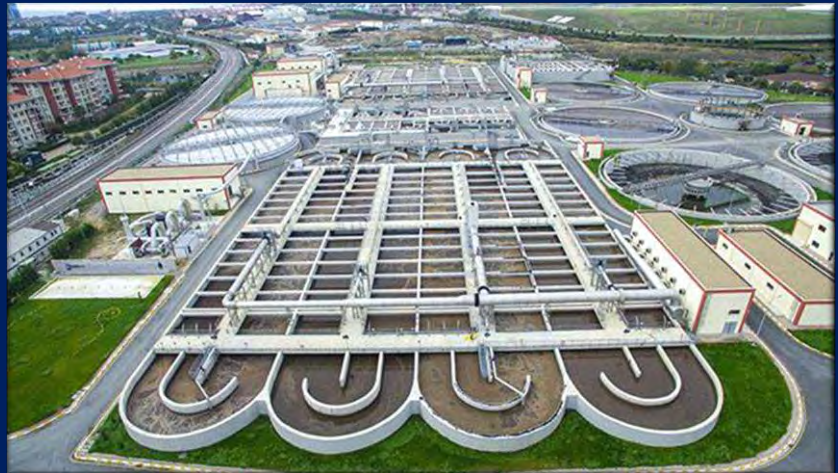
Atakoy Wastewater Reuse Plant – Istanbul, Türkiye.
