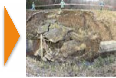
Reservoir embankment restored to original condition damaged again by heavy rain
