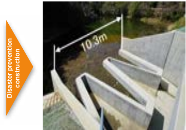
Image of measures against heavy rain (repair of flood spillway)
