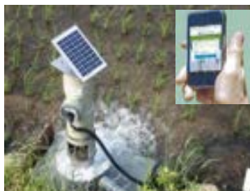
Installation of automatic water taps
