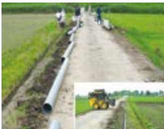
Conversion of open waterways to pipelines
