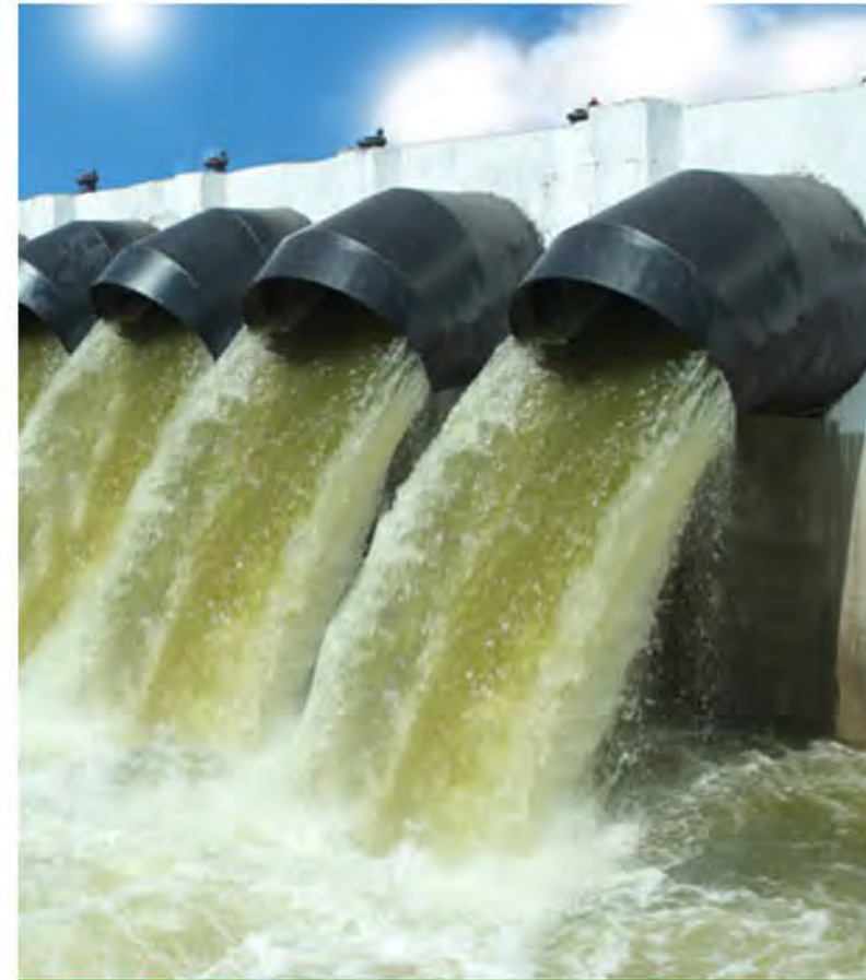
Lift Irrigation Systems
