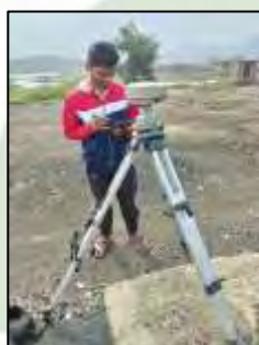
Static DGPS Survey In Progress
